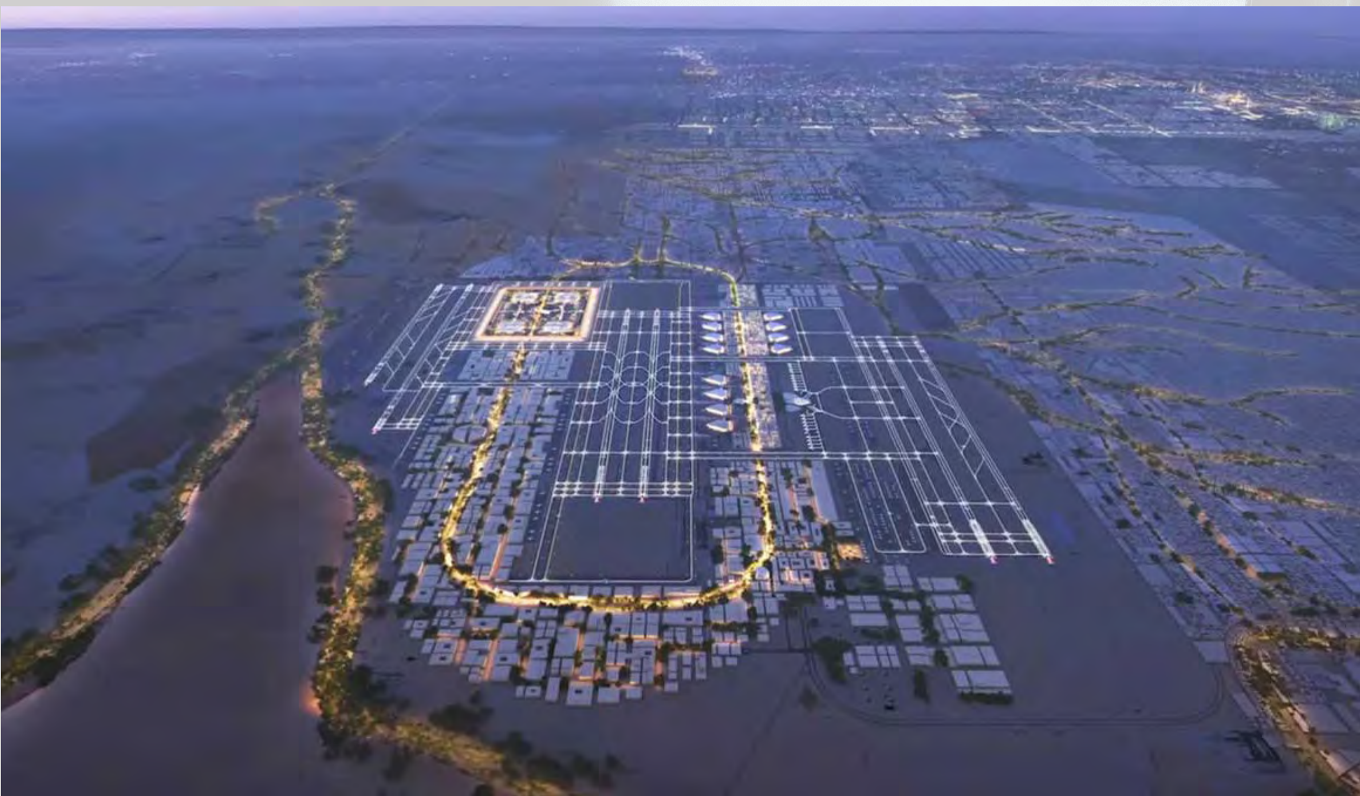
Aerial view of King Salman International Airport in Riyadh (Saudi Arabia).
