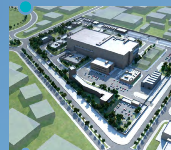
FCC Construcción to build Spain's first particle acceleration experimentation center
