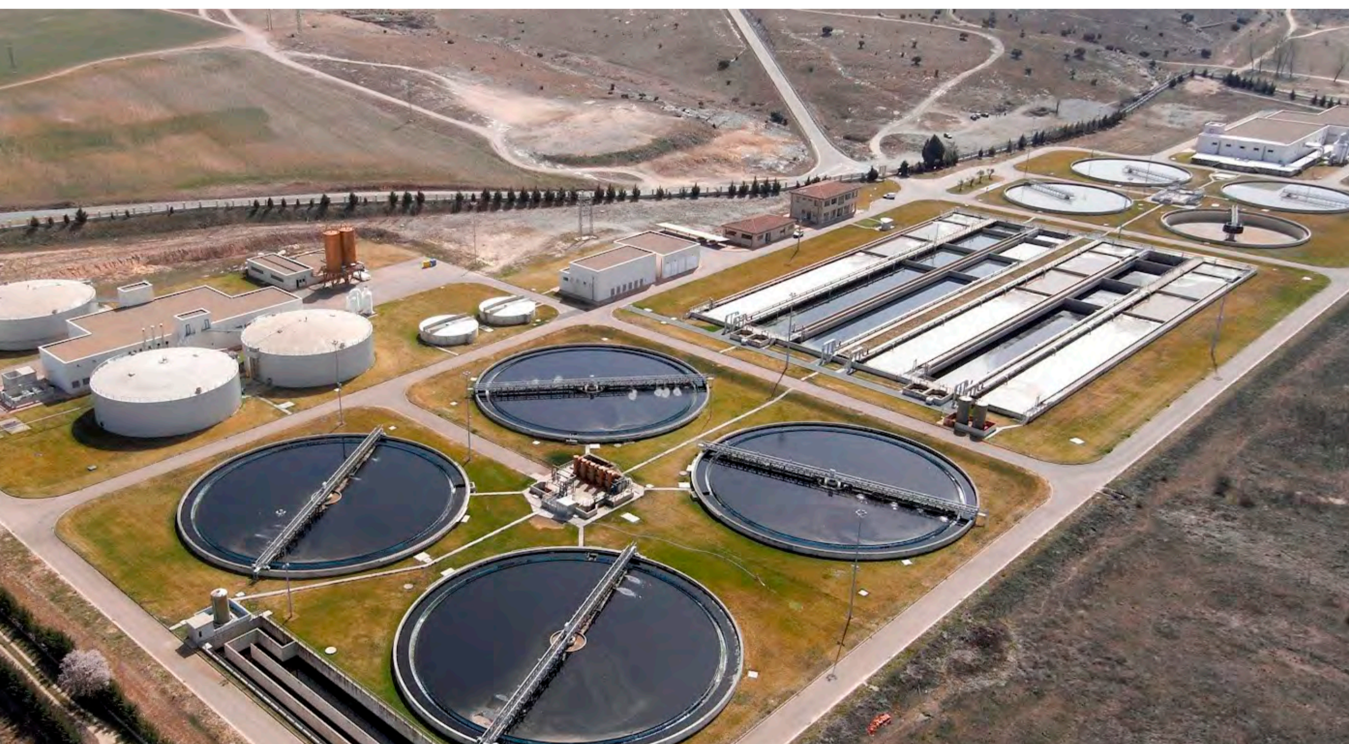
Salamanca Wastewater Treatment Plant.
