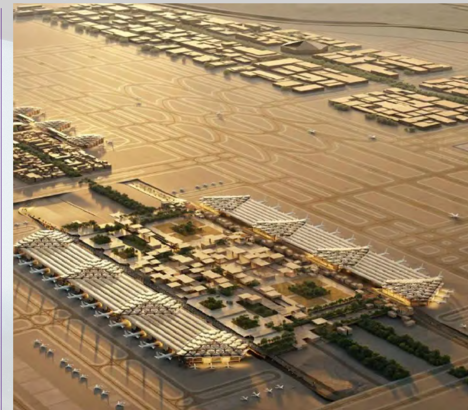
The third runway incorporates multiple access taxiways to ensure a smooth flow of aircraft.
